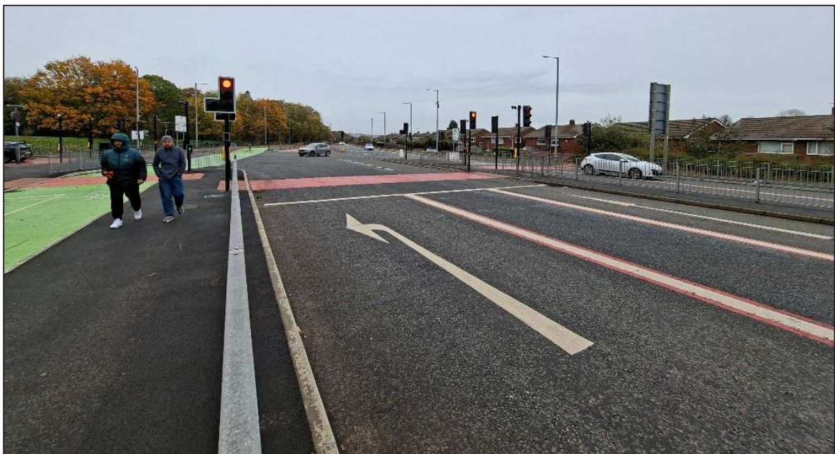
Figure 3.15: B5204 Elton Head Road Junction
