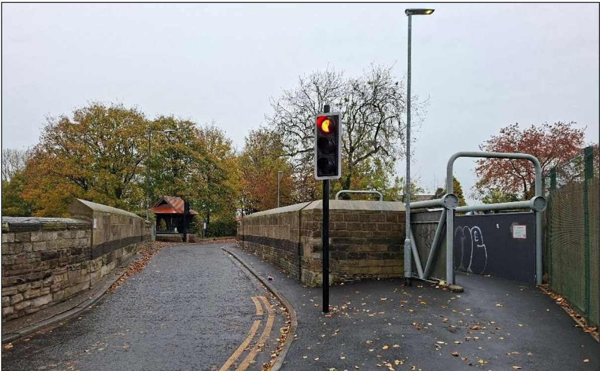
Figure 3.32: New Street – Pedestrian Access to Footbridge
