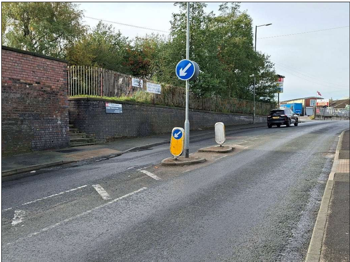
Figure 2.20: Station Road - Refuge Crossing Island
