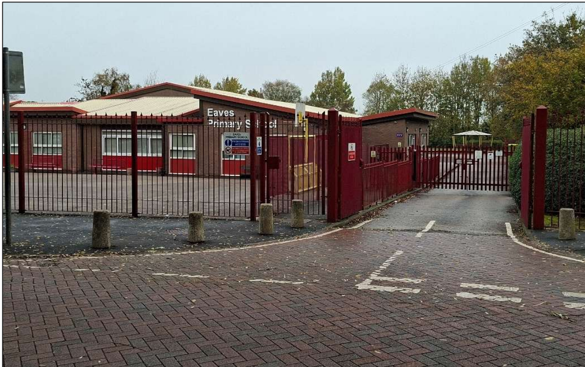
Figure 3.37: Eaves Lane – Eaves Primary School Pedestrian Access
