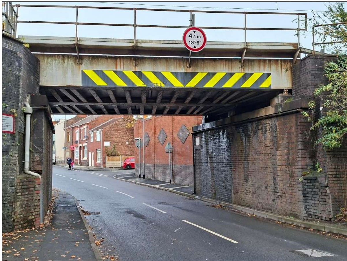
Figure 2.10: Helena Road - Underpass
