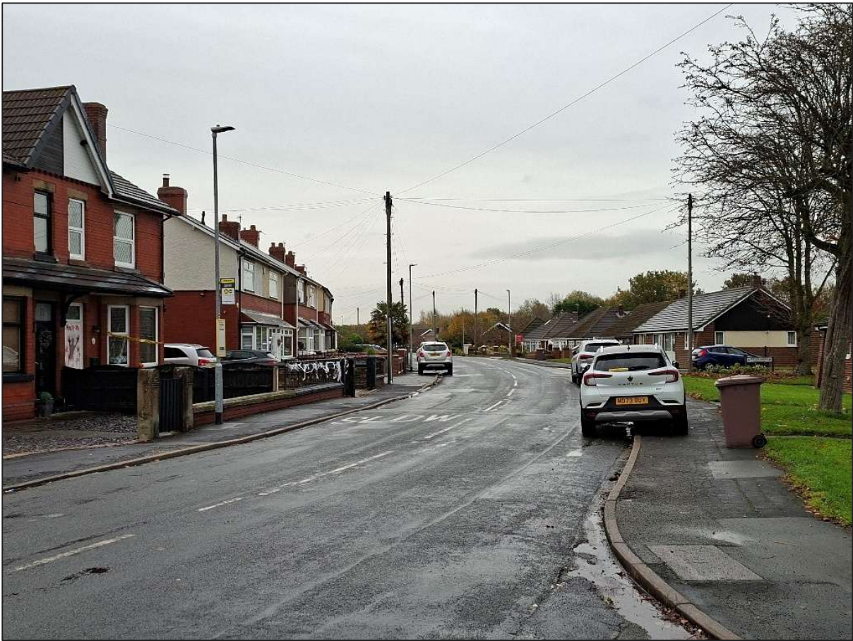
Figure 3.47: Gorsey Lane – Road Markings
