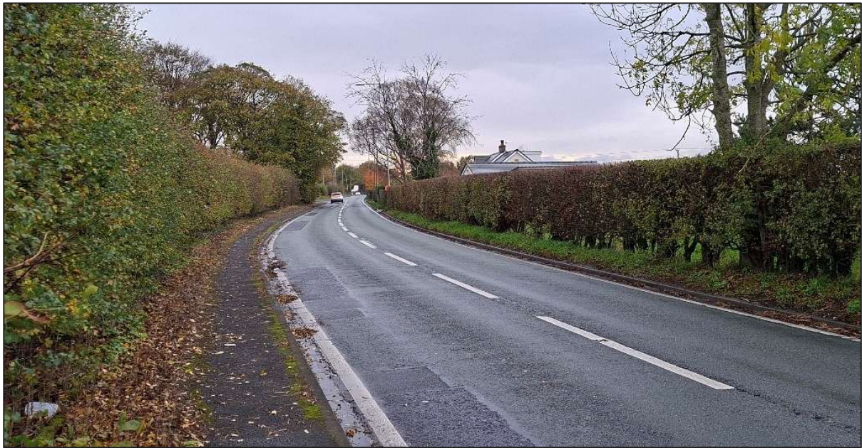
Figure 5.1: Gorsey Lane Western Footway
