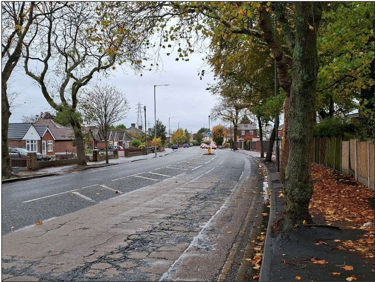
Figure 3.38: A569 Clock Face Road Northbound
