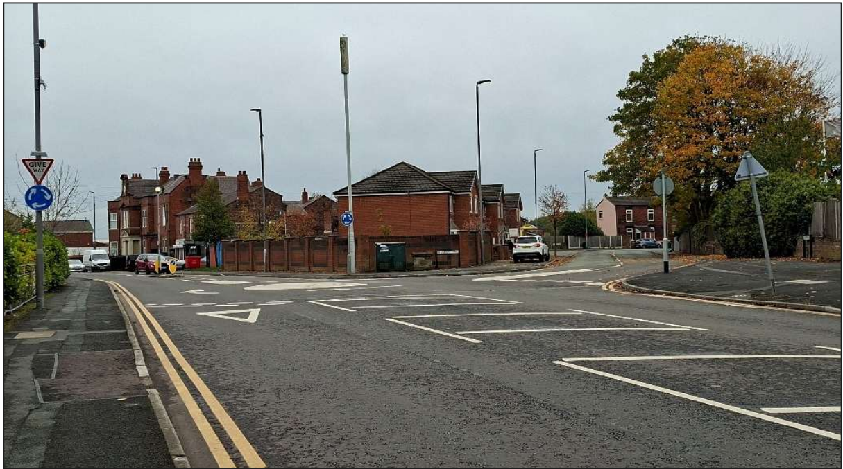
Figure 3.1: Clockface Road / Gartons Lane – Mini Roundabout Junction
