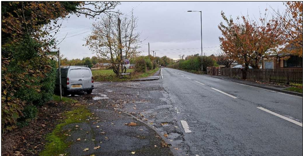
Figure 5.2: Gorsey Lane Junction
