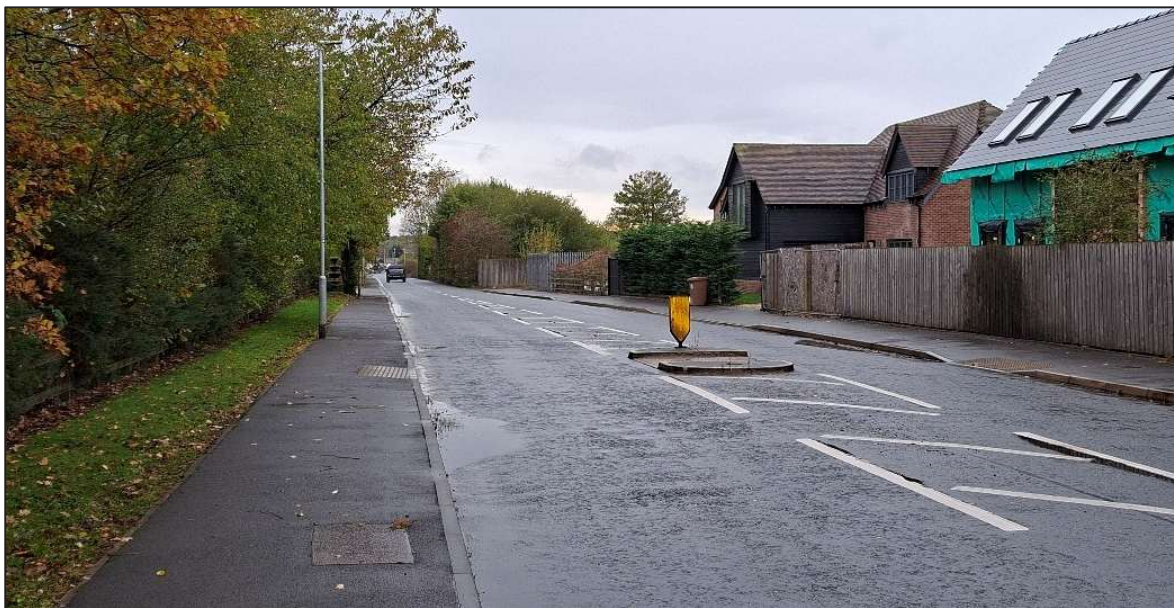
Figure 5.4: Gorsey Lane Refuge Island
