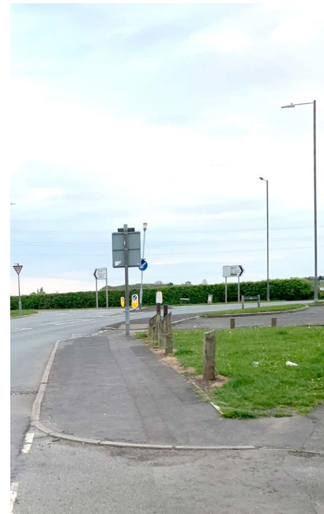
Figure 5.10 The existing junction at Reginald Road / Helena Road that will become a key link from the site towards St Helens Junction Rail Station
