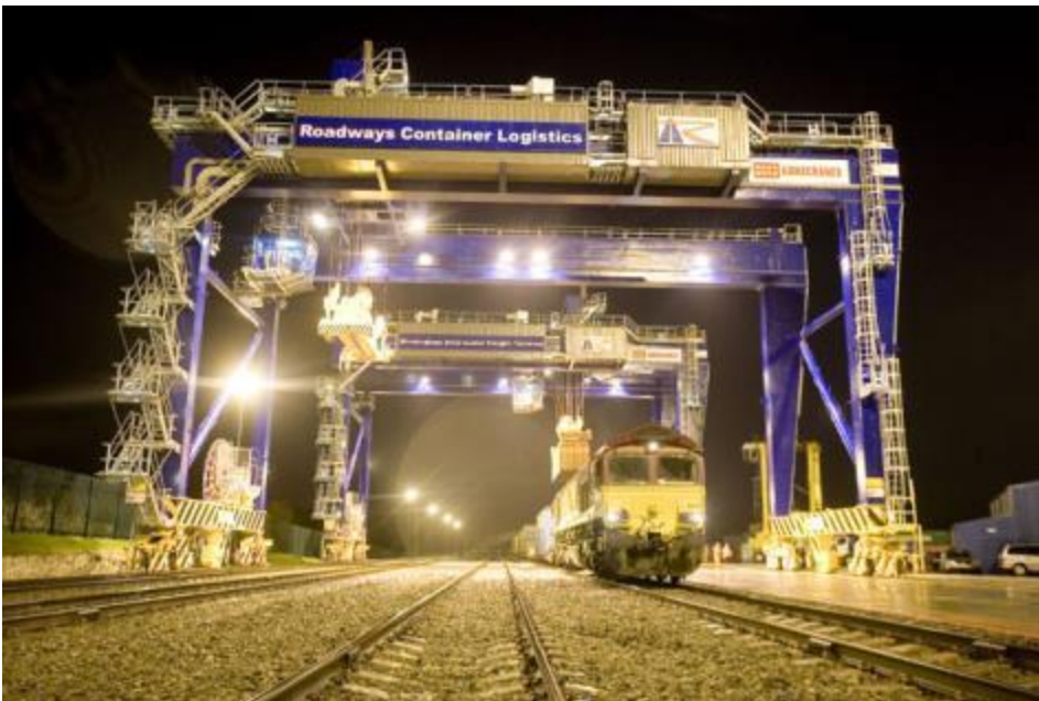
Figure 4.1- Birmingham International Freight Terminal (BIFT)
