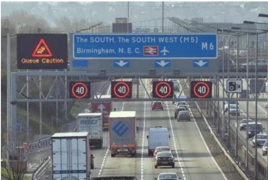
Figure 6.3 – Super Span Gantry on the M6 near Birmingham
