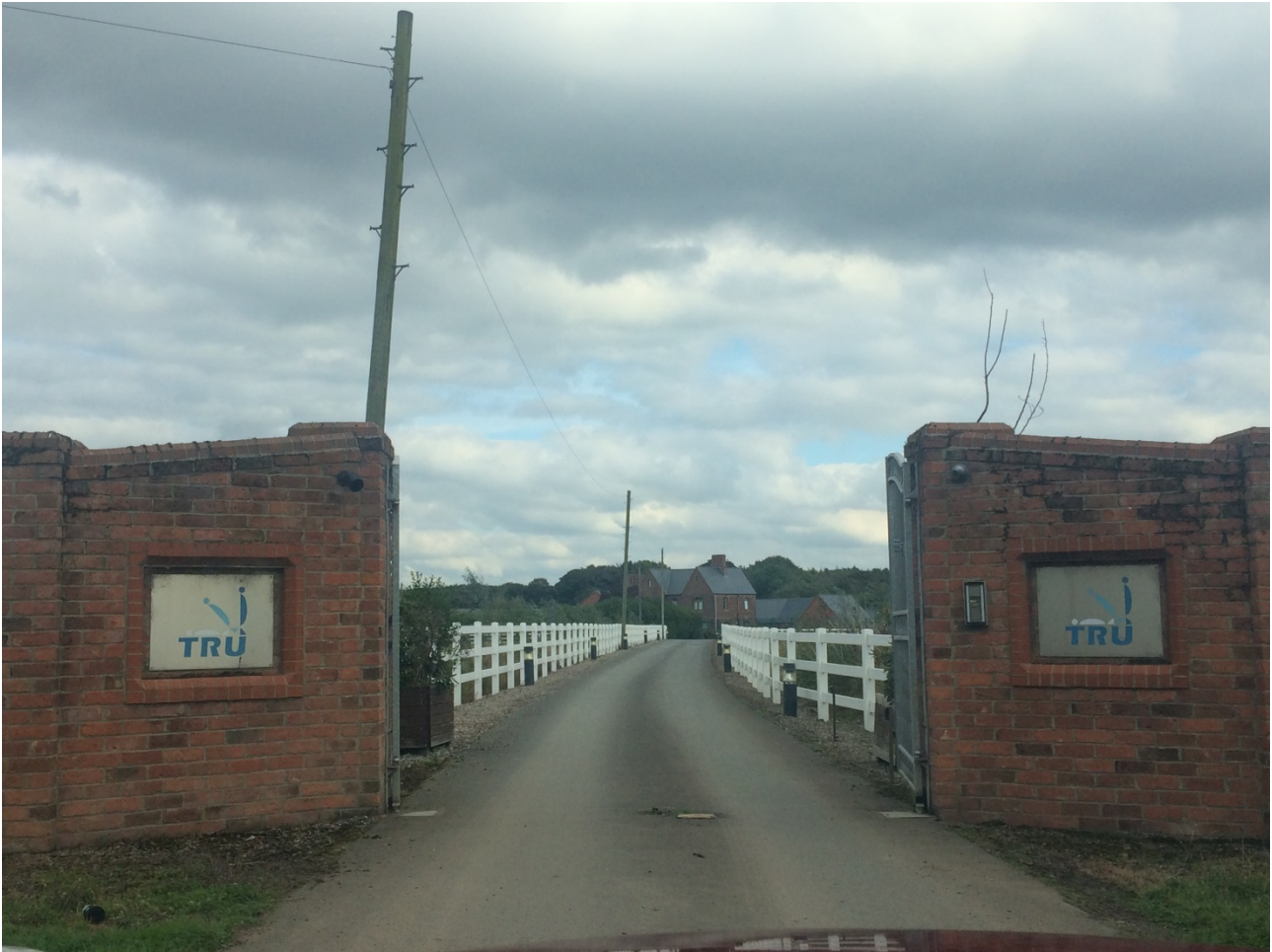
View of the development which currently exists on site
