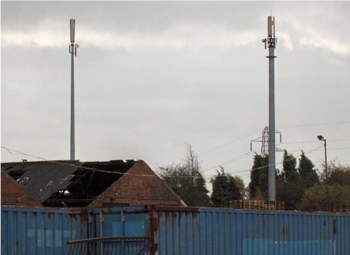
Picture 6.2 An example of using two smaller masts to reduce visual intrusion
