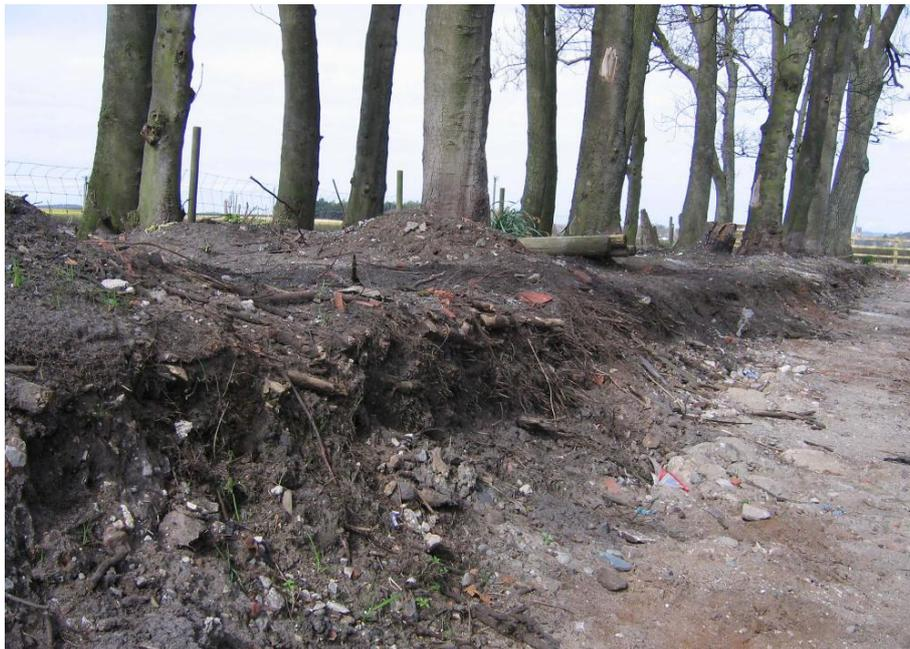
**Picture 5.2 Excavation of roots can lead to the death of trees.**
