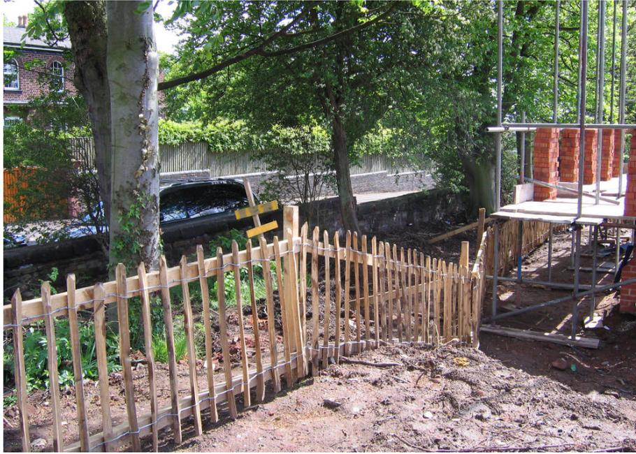
**Picture 5.3 Chestnut paling fencing can be used to secure areas of tree protection**
