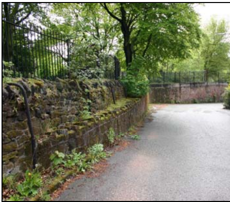
Image 6.2: Holme Road retaining wall
