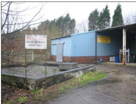
Image 3.7: Demolished Utility Buildings
