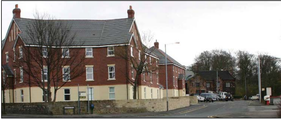
Image 6.1: View along Holme Road from Millfields towards Home Farm
