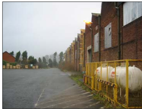
Image 3.6: Demolished Factory Building
