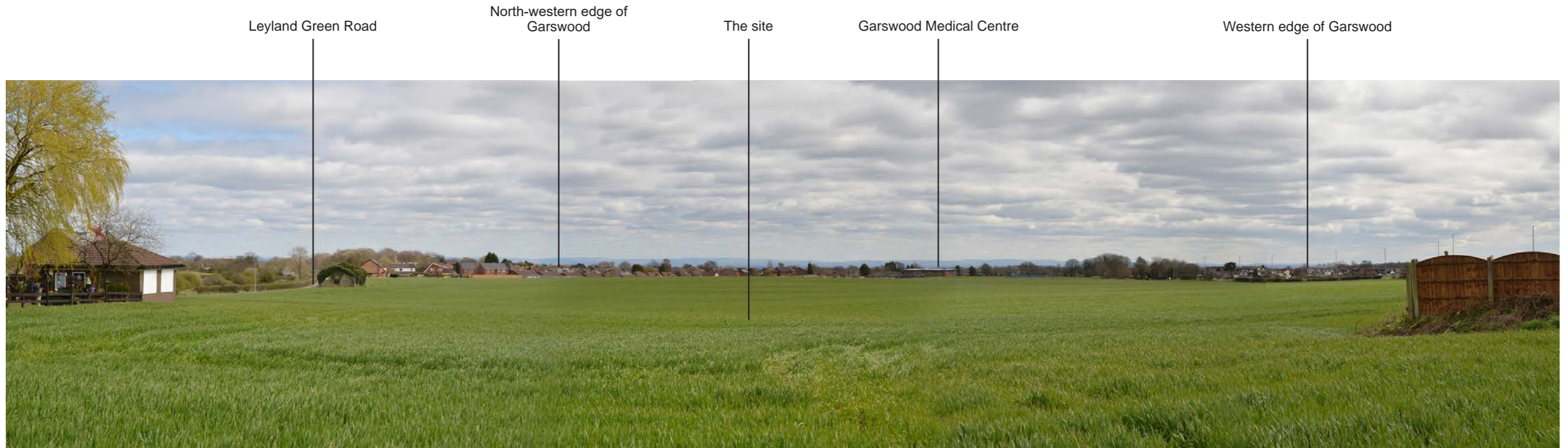
Photograph 6 - Looking across the site from a gap in the ribbon development lining Garswood Road.
