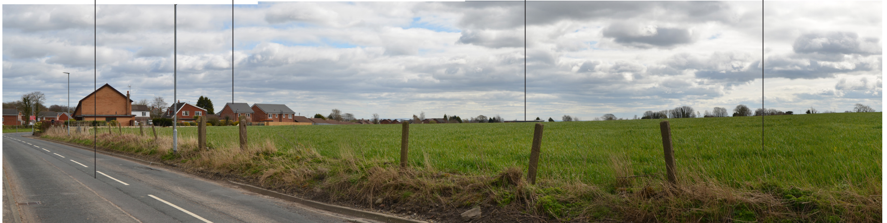
Photograph 5 - View across the site from Leyland Green Road
