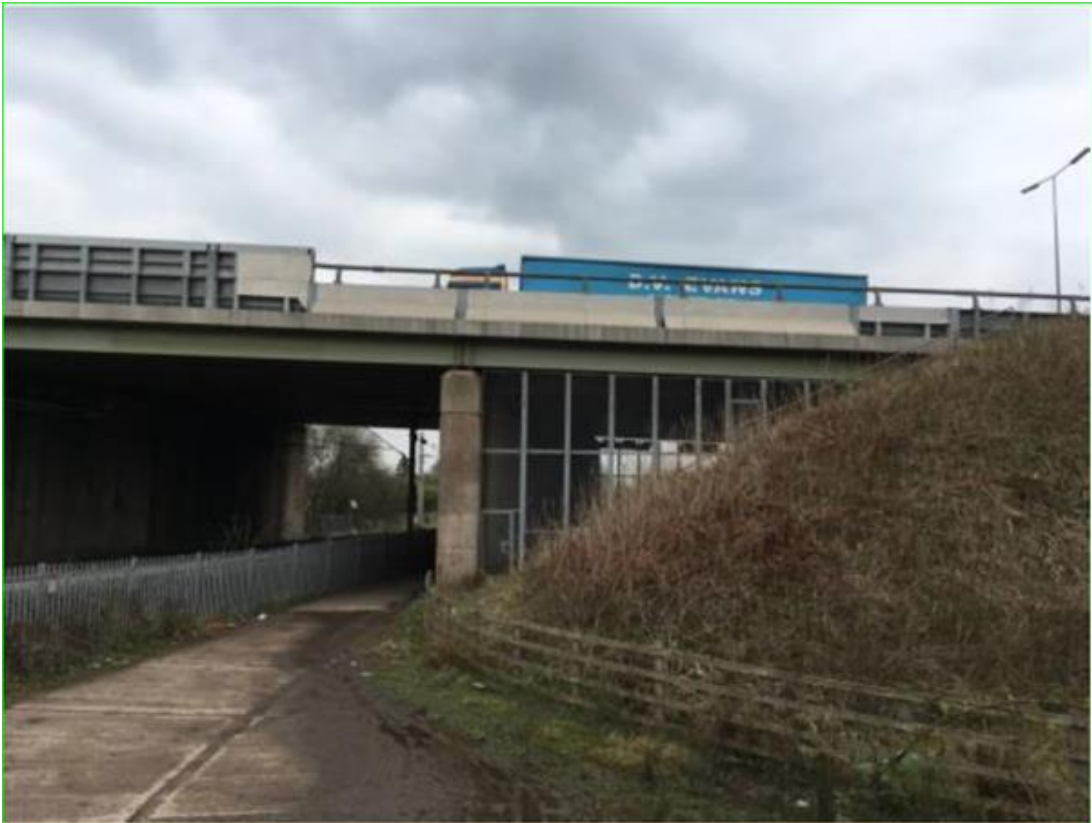
Figure 6 Access Track Running Next to Chat Moss Line
