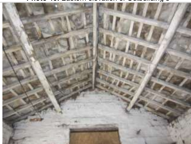
Photo 48: Exposed roof at Outbuilding 5
