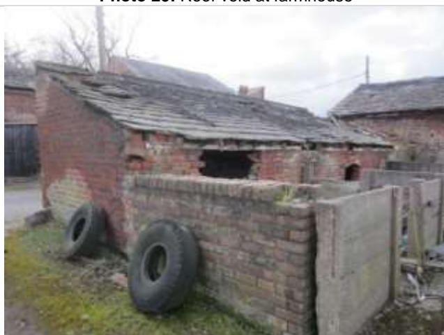
Photo 27: Northern elevation of Outbuilding 1, Section 1a
