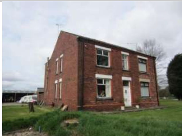
Photo 20: Eastern elevation of farmhouse
