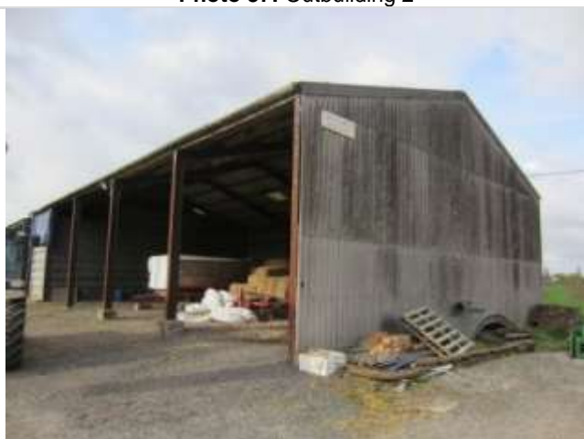
Photo 39: Northern elevation of Outbuilding 2
