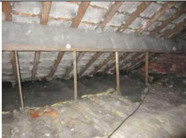
Photo 25: Roof void at farmhouse
