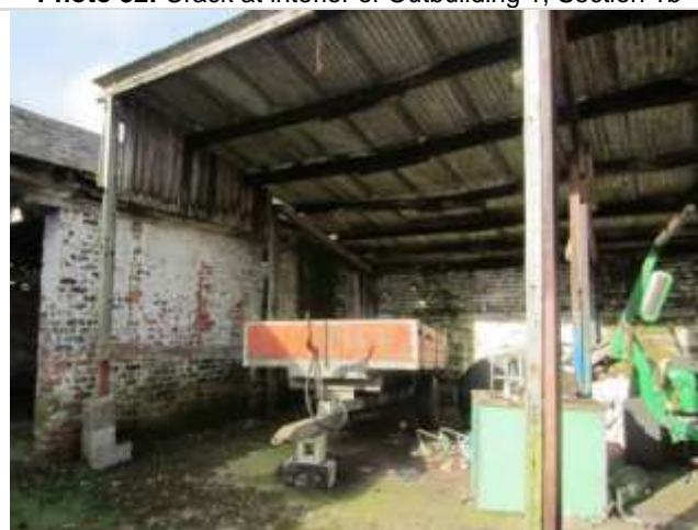
Photo 34: Outbuilding 1, Section 1c
