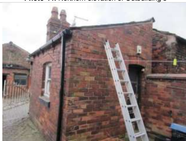
Photo 46: Eastern elevation of Outbuilding 5
