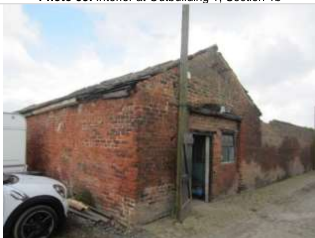
Photo 35: Eastern elevation of Outbuilding 1, Section 1d
