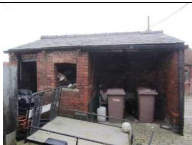
Photo 50: Eastern elevation of Outbuilding 6
