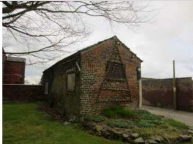
Photo 44: Northern elevation of Outbuilding 5
