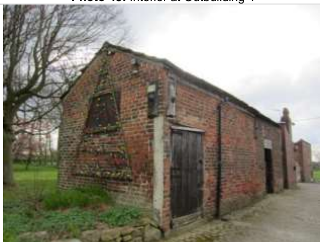
Photo 45: Northern and western elevation of Outbuilding 5
