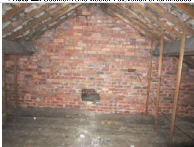
Photo 24: Roof void at farmhouse
