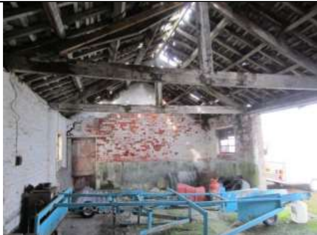
Photo 31: Interior at Outbuilding 1, Section 1b
