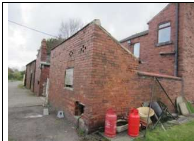
Photo 49: Southern and western elevation of Outbuilding 6
