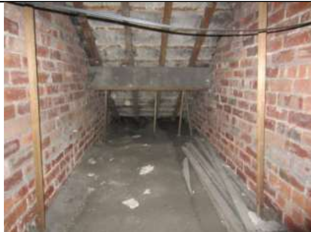
Photo 26: Roof void at farmhouse
