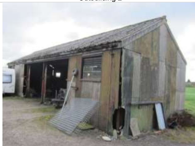
Photo 42: Southern and western elevation of Outbuilding 4
