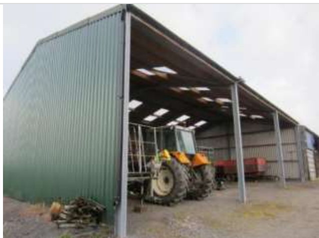
Photo 41: Southern and eastern elevations of Outbuilding 3
