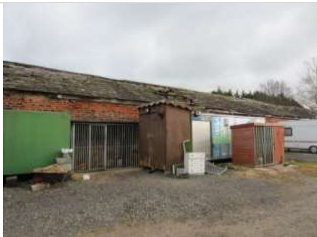
Photo 29: Outbuilding 1, Section 1b
