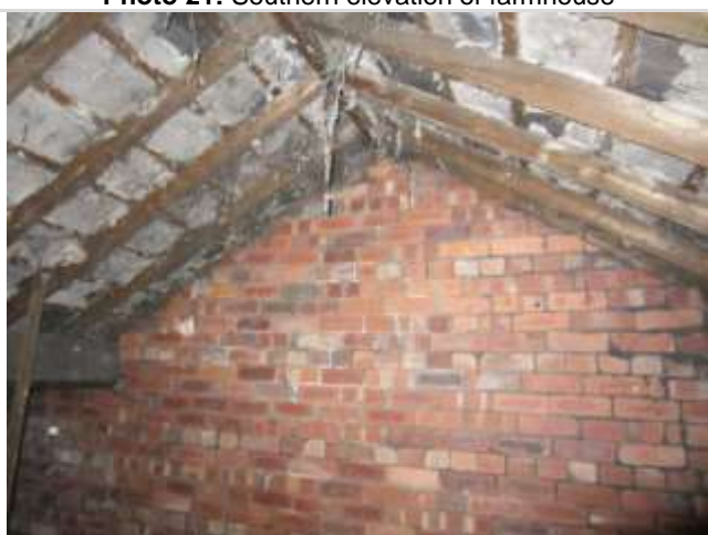
Photo 23: Roof void at farmhouse
