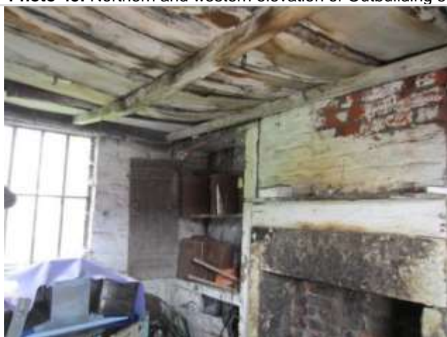
Photo 47: Interior of Outbuilding 5
