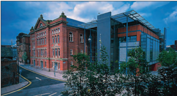
Example of a sensitive extension to a Listed Building, Victoria Hall, Stoke.
