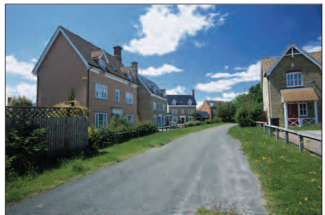
Example of a frontage with a deep set back from the street.
