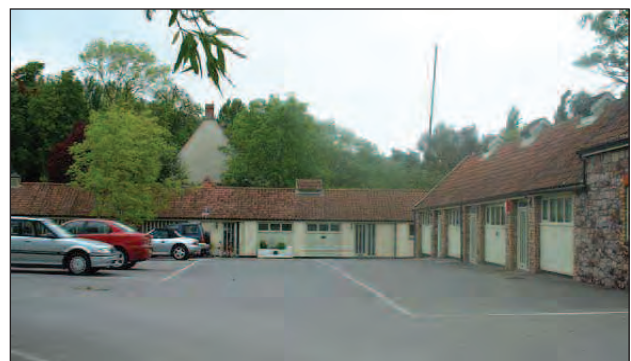
Business units created by conversion of outbuildings.
