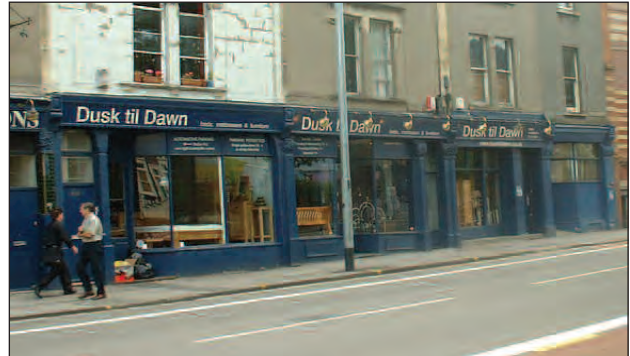
Example of a shopfront which extends over several properties, at the same time retaining the integrity of the individual bays, and traditional features.
