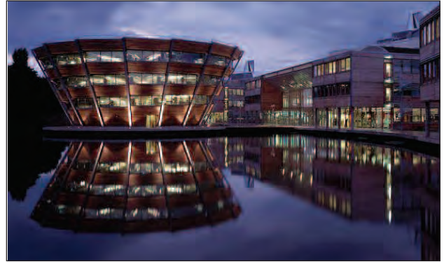
Jubilee Campus, Nottingham University. The requirement to incorporate environmentally friendly technology and materials was a requirement from the outset, and this ensured that there was no impact on capital costs.
