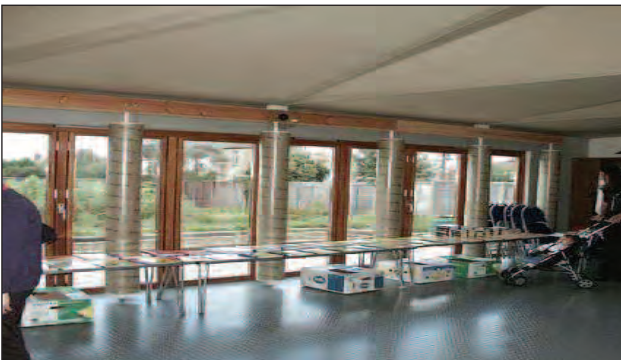
The Cardboard Building, Westborough Primary School, Westcliffe on Sea is made of cardboard and timber with 90% of the materials being recycled.
