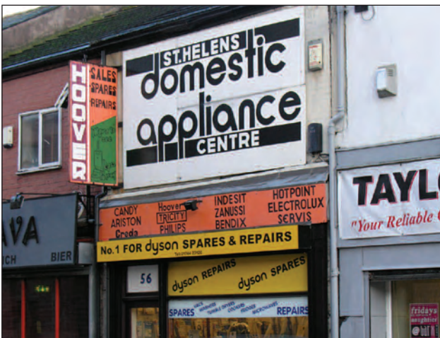
Example of inappropriate signage creating a very cluttered and poor quality frontage to the shop.
