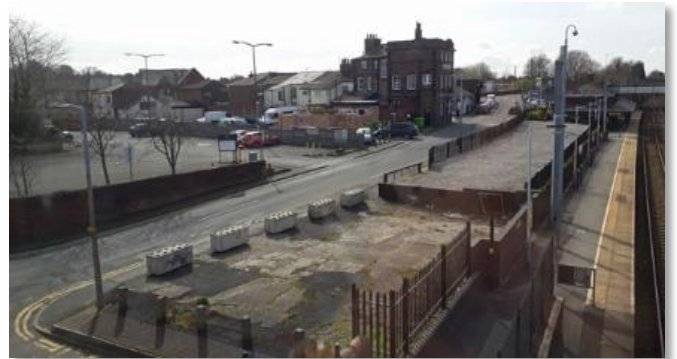
Land adjacent to Rainhill Station, on the village side, viewed from the pedestrian bridge across the track; the Liverpool-bound platform is visible on the right.
