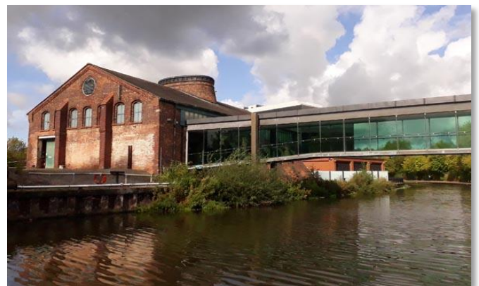
No. 9 Tank House, Pilkington Jubilee Works – now part of The World of Glass
