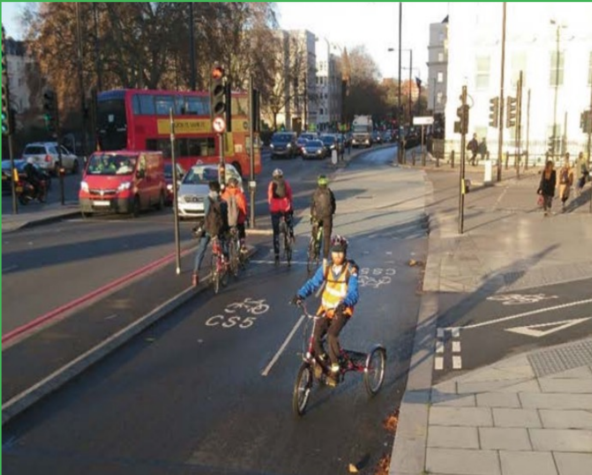
FIGURE 1.1/1: EXAMPLE OF A CARRIAGEWAY-LEVEL CYCLE TRACK WITH CONTINUOUS KERBS TO FOOTWAY AND CARRIAGEWAY, FROM CYCLE INFRASTRUCTURE DESIGN GUIDANCE DOCUMENT (LTN 1/20).
