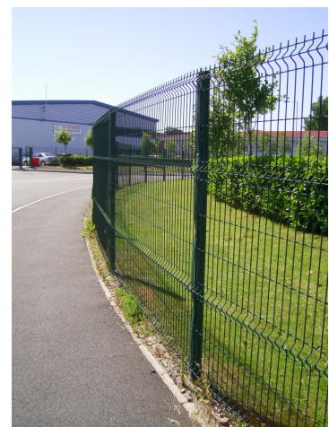
Example of good visibility with a boundary fence on a business park.
