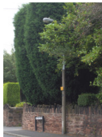
Lighting columns should not be obscured by trees.
