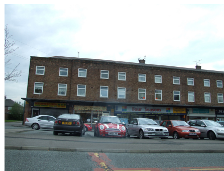
Surface car parking can have a negative effect on street frontages.
