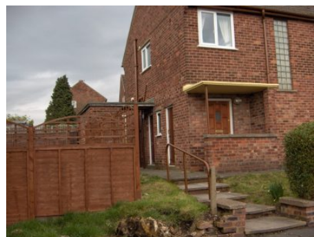
Example of porch roof and side extensions providing opportunities for climbing and access.
