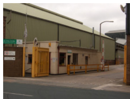
Example of a security point at the entrance to an industrial site.
