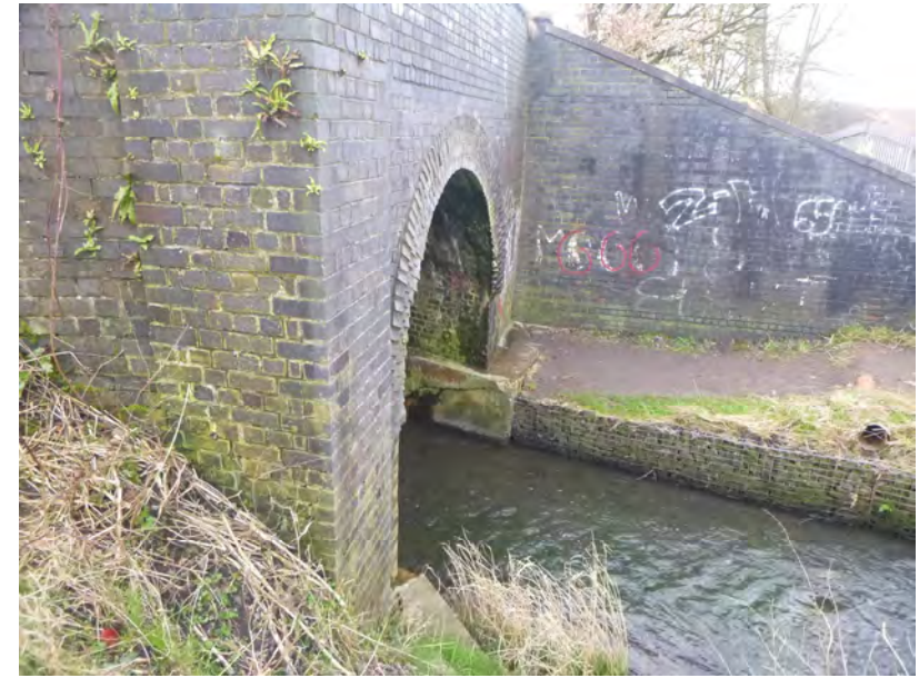
Newton Brook crossing under Railway
